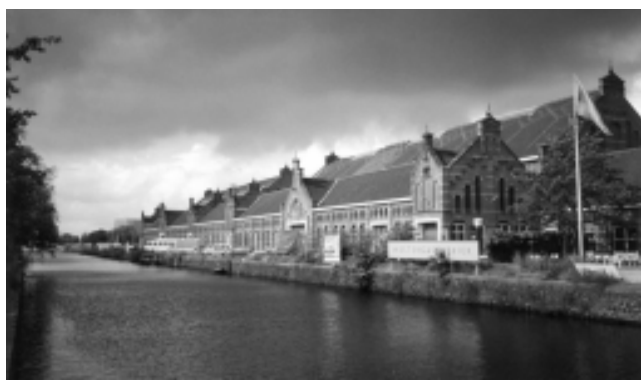
Fig. 5. A polluted MGP site: the 'Westergasfabriek' in Amsterdam, The Netherlands
