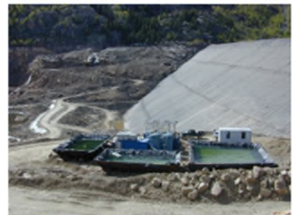
Figure 3. The EC system was set up to treat water that had been used in the manufacturing of a dam. The water was recycled for reuse. Figures 1, 2, and 3 were taken at the Homestake Dam, Colorado.
