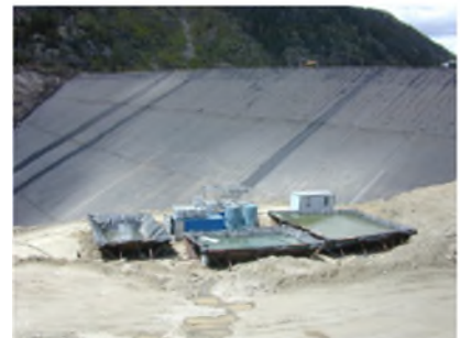
Figure 2. The electrocoagulation system can be set up to remove metals in nonmetallic mine or milling process.
