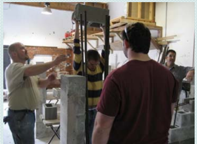
Below: Laying 12" CMU with rebar laps
