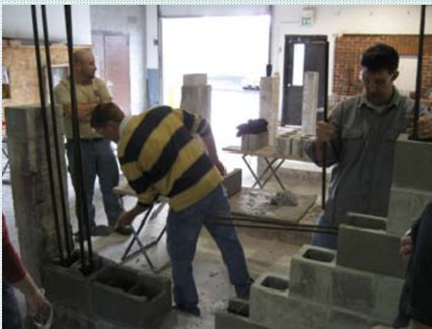
Above: Rebar placement in a CMU wall
