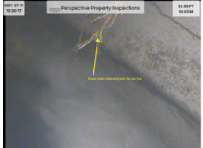
Roots extend into the city sewer line
