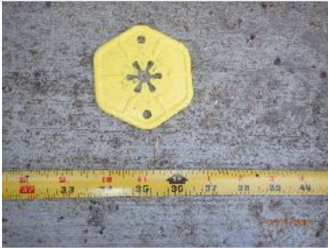
Surface measurements and view of off set and root intrusion
