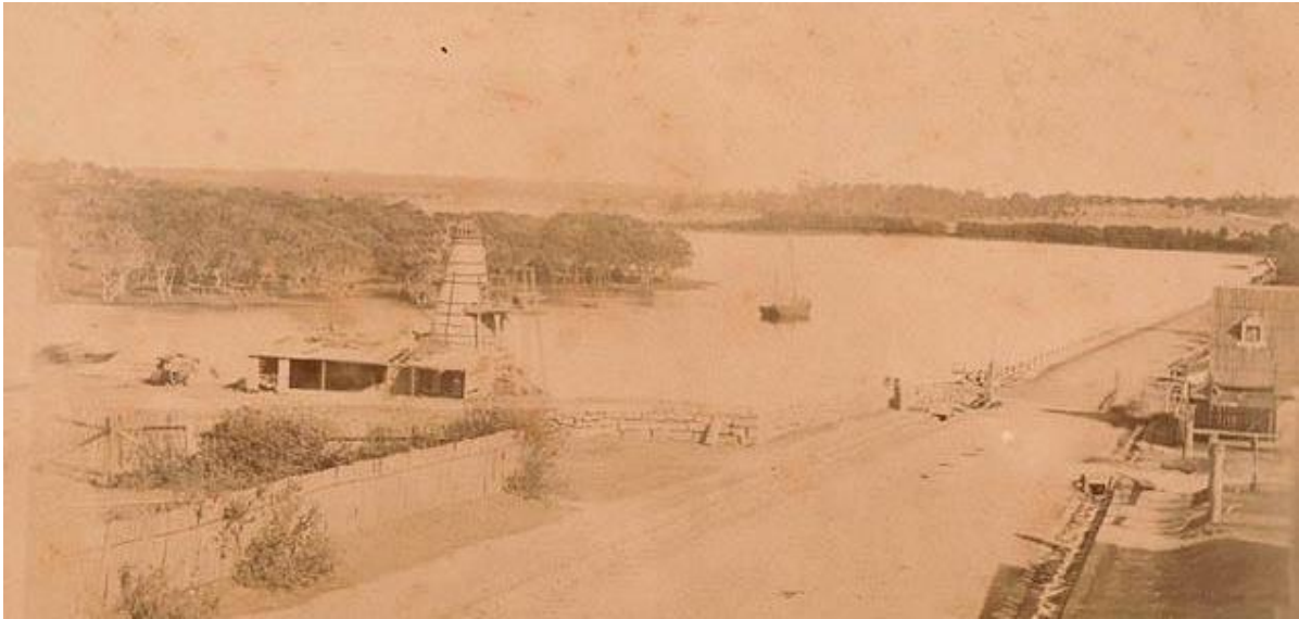
Figure 48. Lime Kiln, Cooks River Dam Tempe. Anonymous. c.1870
