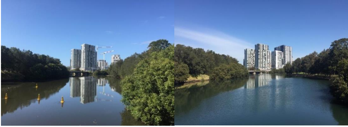
Figure 43. Research image. Construction at Wolli Creek 2017 and 2019.
