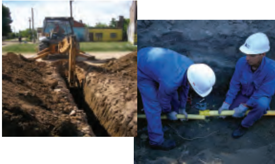
Gas network infrastructure building
