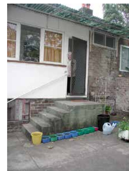
Peggy's rainwater-collection system, 2009
