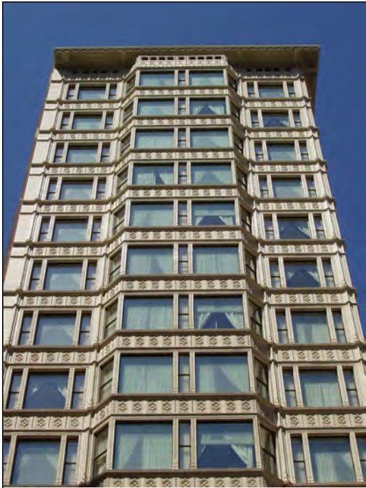
Figure 22. The Reliance building, Chicago
