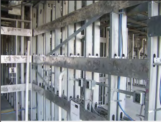
Figure 19. Metal Stud wall
