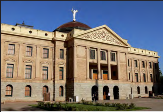
Figure 2. The stern historic Arizona State Capitol
