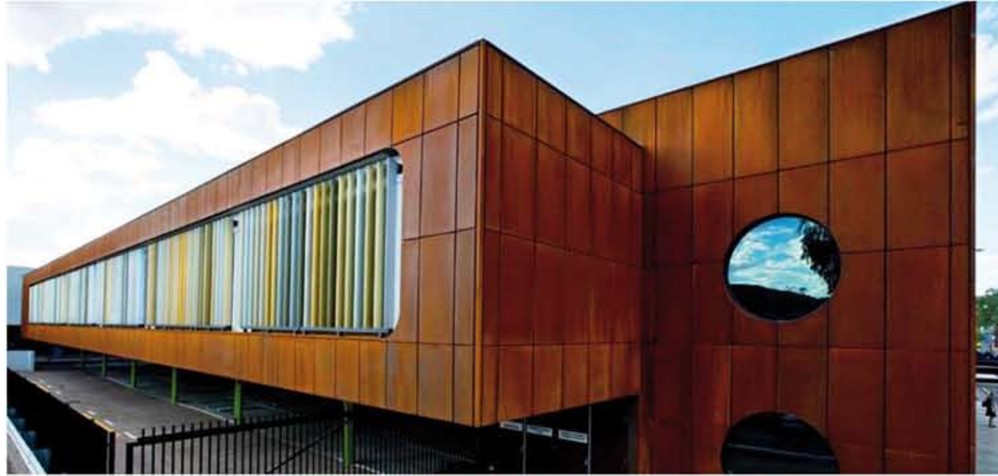
CORTEN A CLADDING (CASSETTE PANELS), ALICE SPRINGS |
