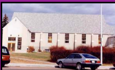
#4: Inglewood CRC pre-renovation (1992 - 2000)
