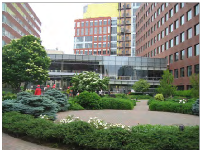
The Google expansion is transforming the former open air passageway from Main Street to the rooftop garden into a small shopping arcade.
