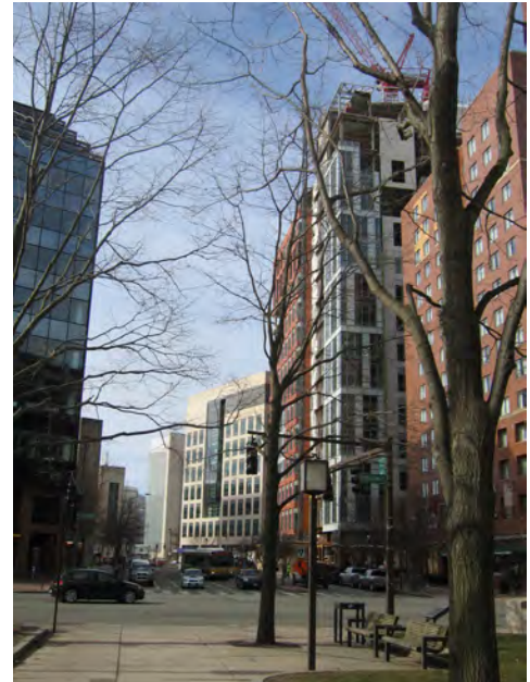
Expansion of the Broad Institute along Ames St shown in the middle. The existing Broad building is to the left of the new building.
