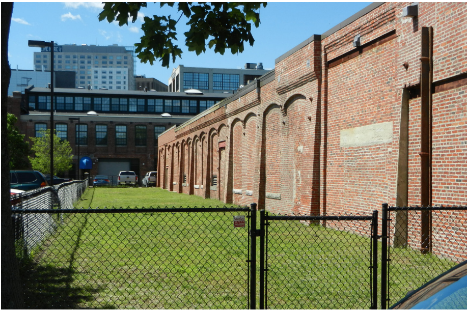
Side yard with view from Bent Street
