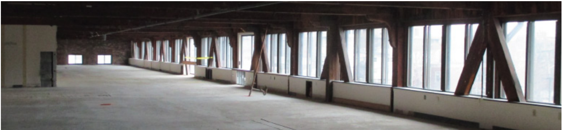
Existing interior space on the 2nd floor
