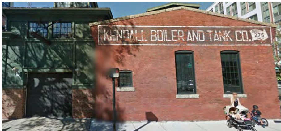
Kendall Boiler and Tank Company Building
