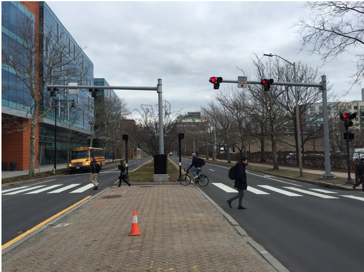
Image F: Existing Conditions at 6th Street Walkway & Binney Street (2017)
