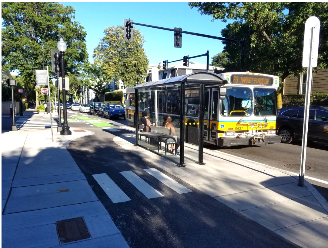
Image C: Example of floating bus stop used on Western Ave with a City-owned and maintained Daytech shelter
