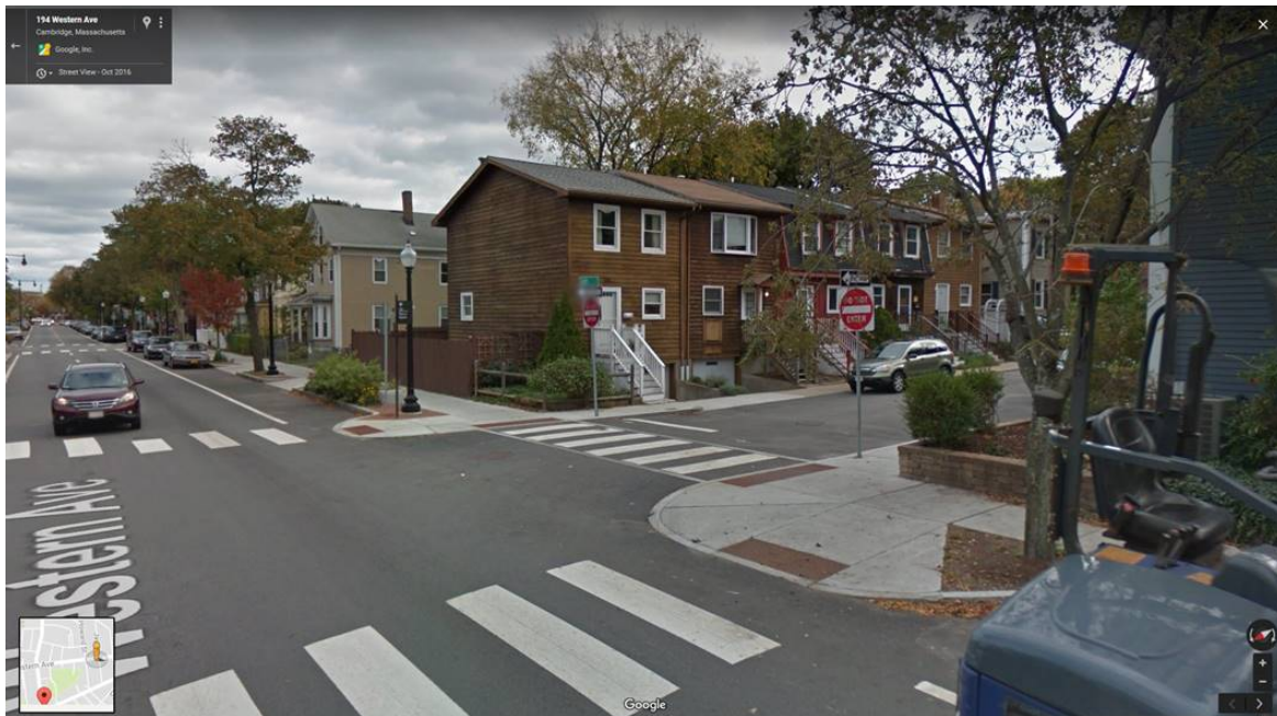
Image I: Example of a Cambridge Modified Raised Crosswalk on Western Ave
