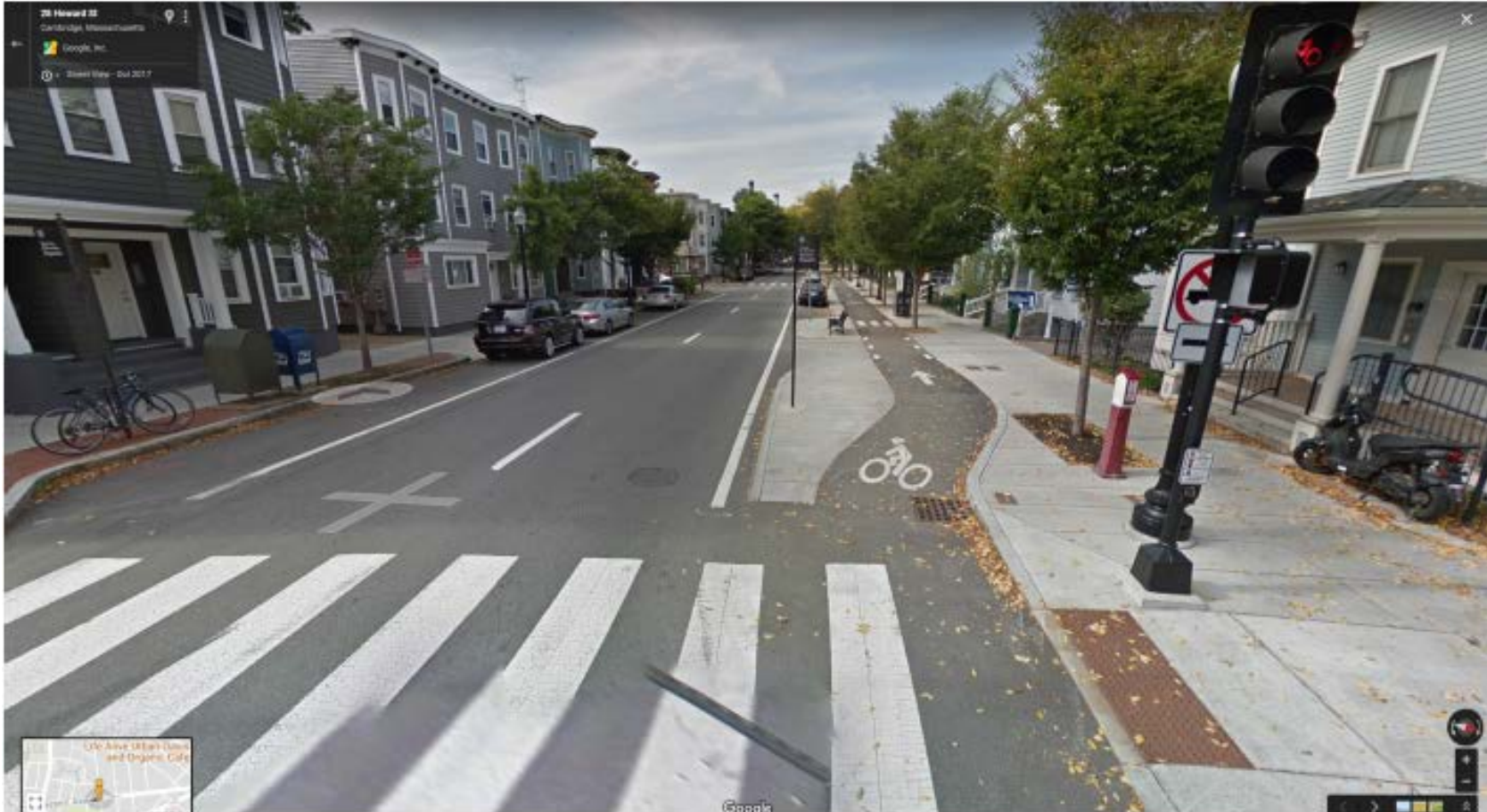
Image E: City of Cambridge's preferred separated bike lane transition as seen on Western Avenue
