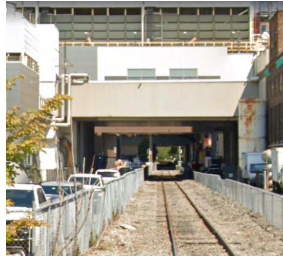
Figure 44. View from Massachusetts Avenue Looking North towards the MIT Co-generation Plant, Which Spans over the Existing Track
