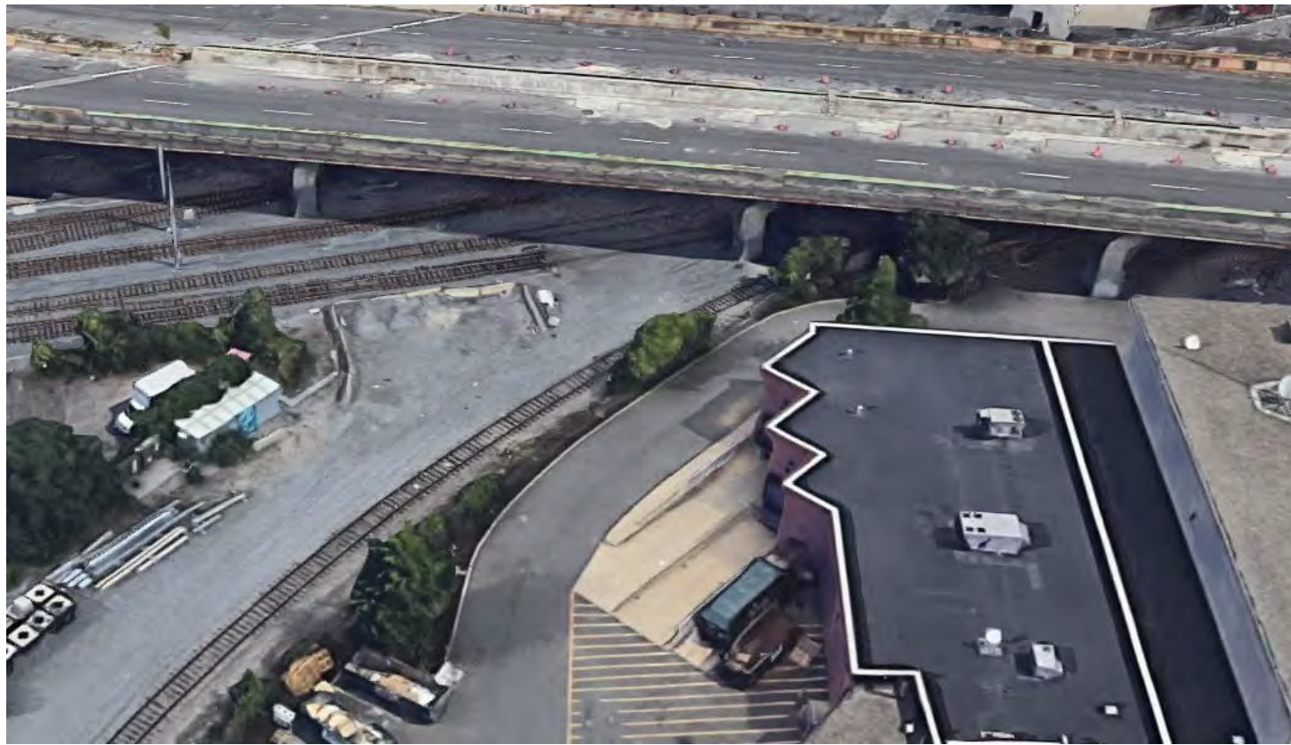
Figure 6. McGrath Highway Support Column Presents an Obstacle to Double-track Extension towards North Station (Source: Google)
