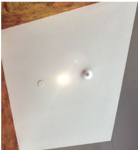
Interior wall angles
