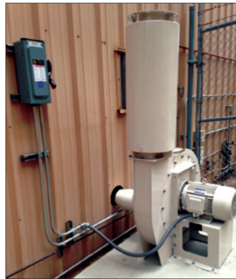
Figure 6. Installation of cooling blower external to laboratory space.
