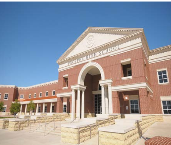
Prosper High School New High School and Indoor Practice Facility Prosper Independent School District
