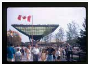
Site 1: Sevihcra Project, Expo67
