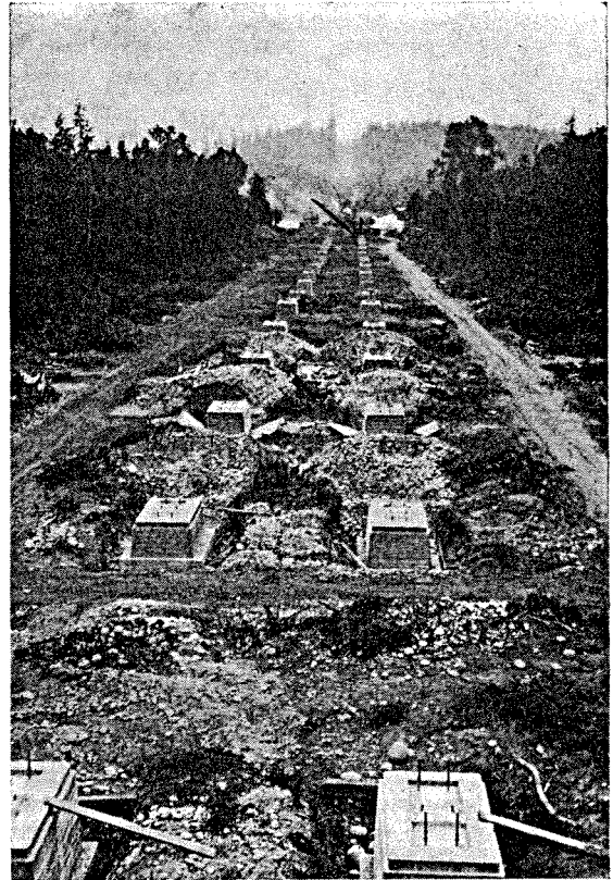
Fig. 18—Pedestals for north viaduct.
