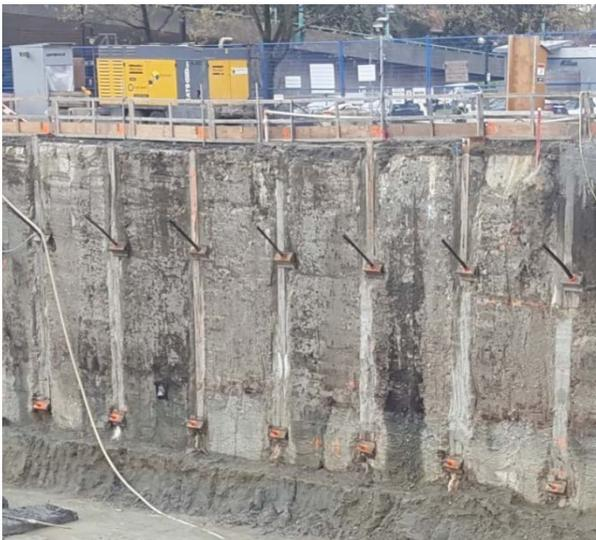
**Fig. 9.** Shotcrete lagging installation below CSM panel at Hybrid Shoring Wall 1
