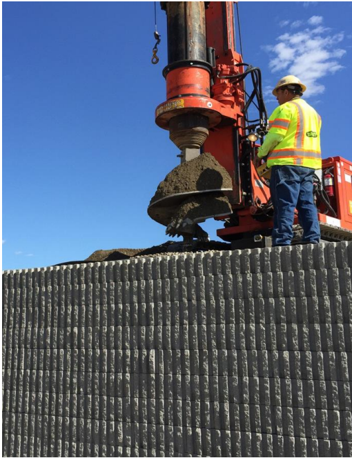
Fig. 6. Drilling after MSE Wall Construction with Rock Auger
