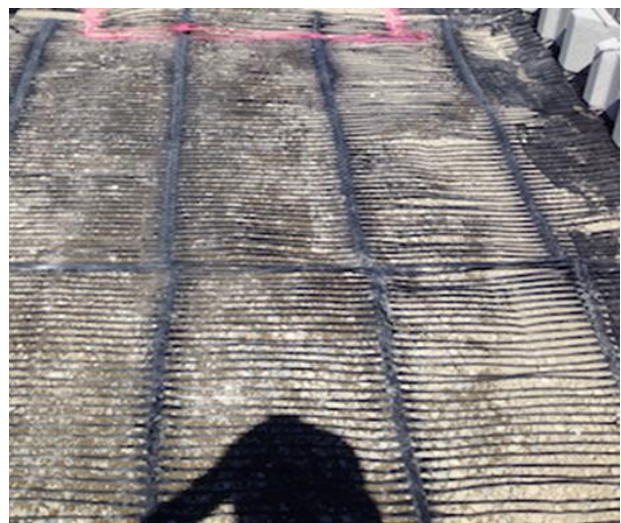
Fig. 3b. No Precut Geogrid Installation
