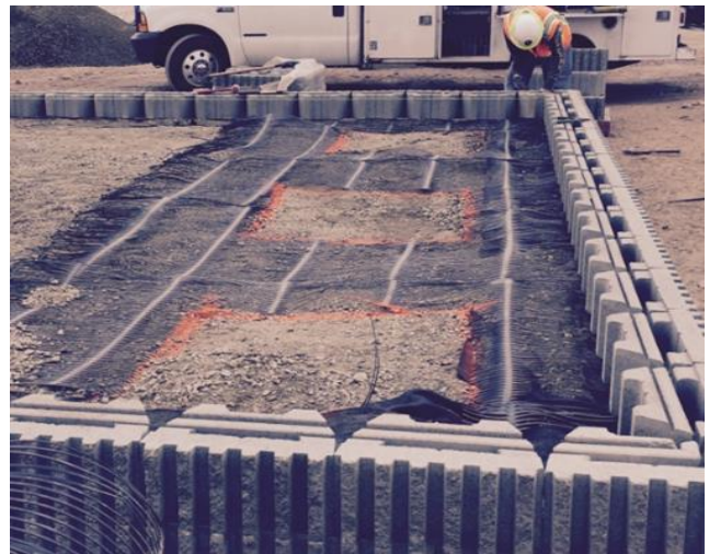
Fig. 3a. Precut Geogrid Around Bore Hole
