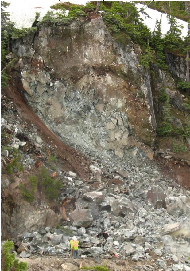
Figure 4 - Final face and blast pile
