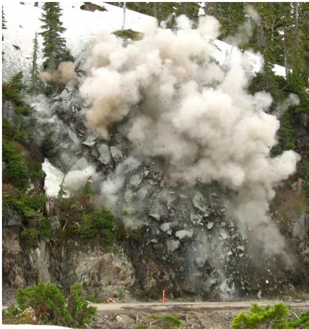
Figure 3 - Photograph mid blast showing good fragmentation
