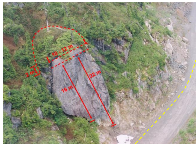
Figure 2 - Aerial Photo of the shield – Yellow dashed line shows centre line of the penstock
