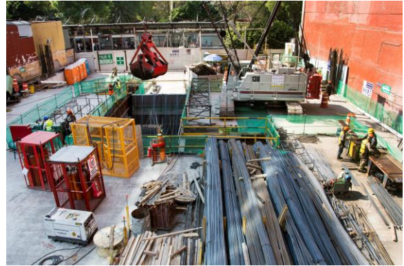
Fig. 19. Working platform slab for Top-Down.
