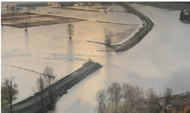
Fig 3. Aerial image of the dike breach.
