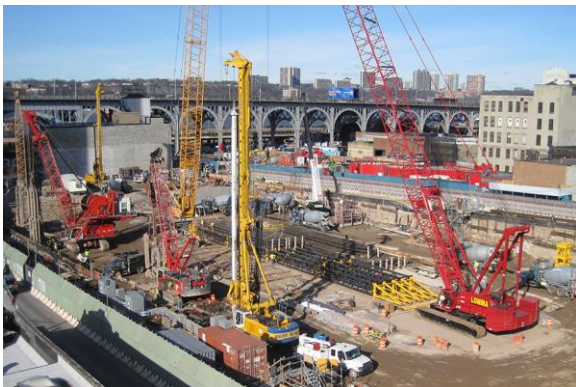
Fig. 28. D-Wall and Pile works for Top-Down.
