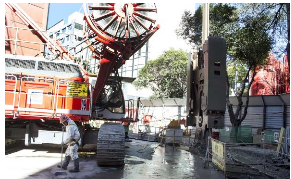
Fig. 12. Hydraulic grab excavating a D-Wall panel.
