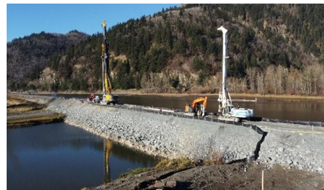
Fig 15. CSM and pre-drilling equipment.
