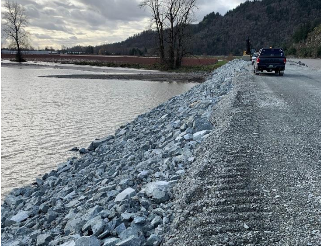
Fig 8. Landside slope of the completed dike breach closure.
