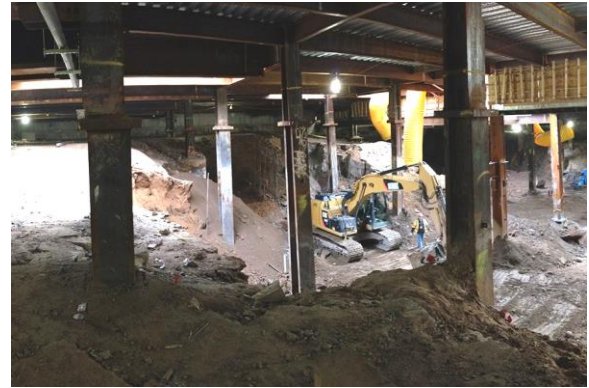
Fig. 29. Under slab Top-Down excavation.
