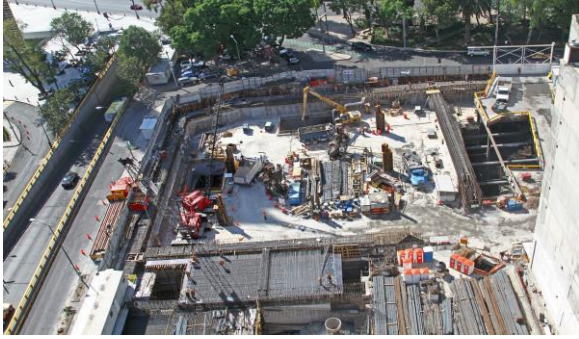
Fig. 22. Civil works and under slab excavation.
