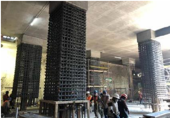
Fig. 9. Definitive columns built while excavating.
