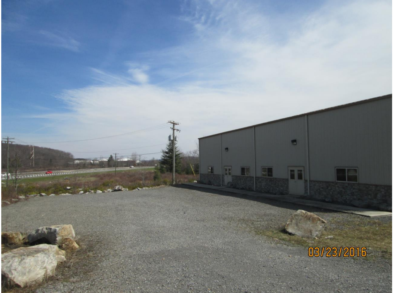
Front Entrance, Corridor H adjacent
