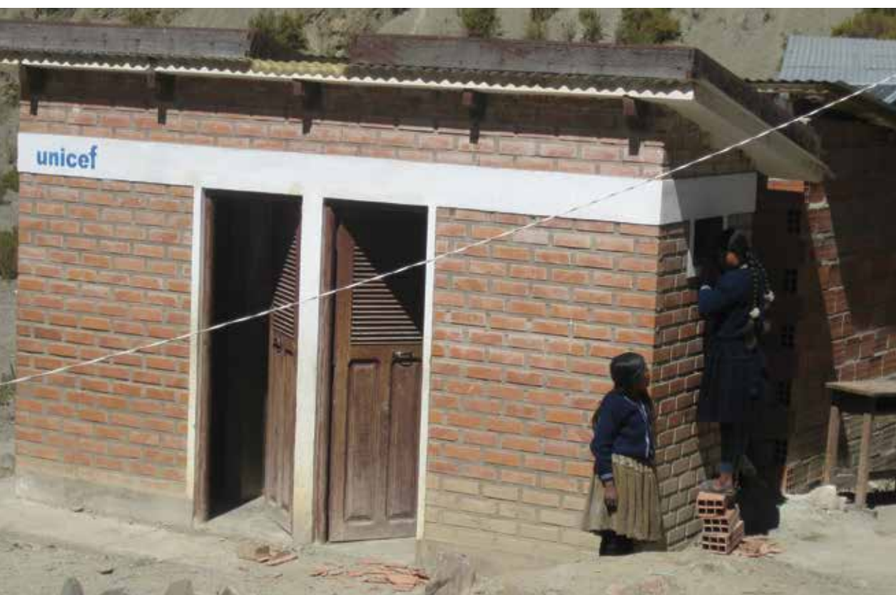
Girls play at broken showers, constructed by the municipality with UNICEF support. Lack of maintenance is an overarching issue for WASH facilities in schools.
