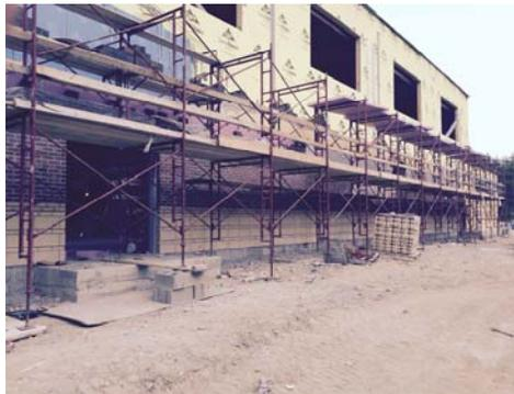
The construction phase of Mildred L. Day is proceeding at a good pace. The building shell is weather tight with windows and roofing intact. Mechanical and electrical trades are roughing in their systems and the masons have completed the block and brickwork. Additionally, the classroom
