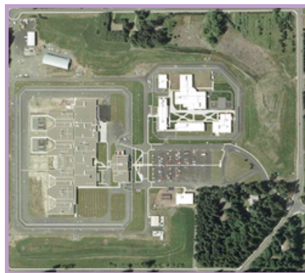
Aerial view of Coffee Creek Correctional Facility. Source: US Geological Survey "The National Map" 85
