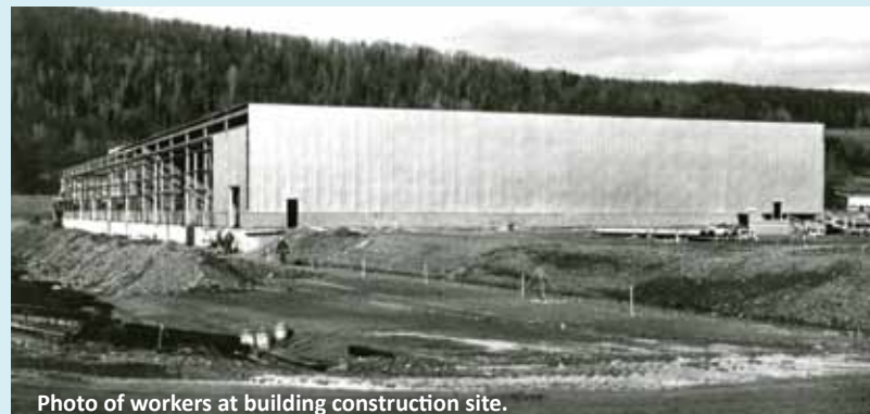
Photo of workers at building construction site.
