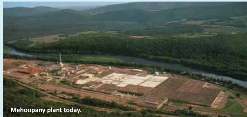
Mehoopany plant today.
