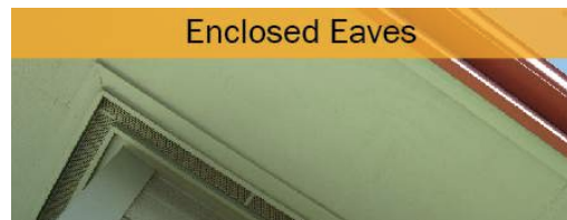
Figure 36. Make sure your eaves are enclosed with non-combustible materials to prevent ember entry.
