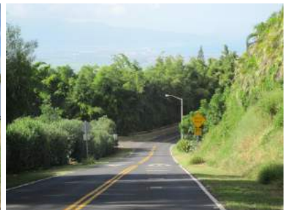
Heavy, hazardous unmanaged roadside fuels
