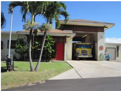
Makawao Fire Station
