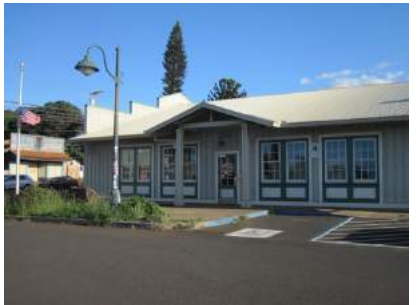
Hazardous fuels near post office
