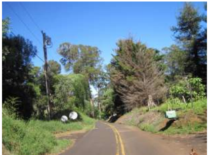
Wildfire hazards along roadside and on telephone poles
