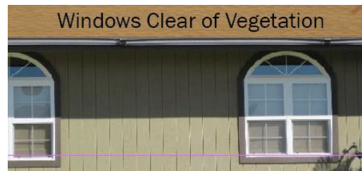
Figure 13. Keep windows free of vegetation to reduce likelihood of heat-caused breakage that lets embers into your home.
