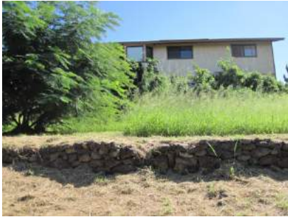
Example of home with hazardous tall grasses and shrubs near windows
