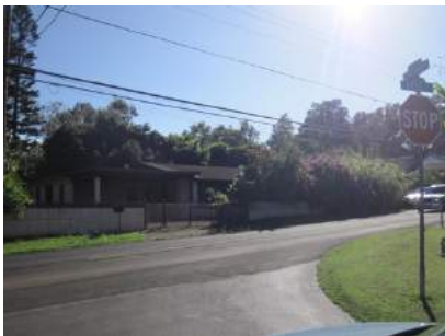
Example of home with hazardous vegetation on fenceline
