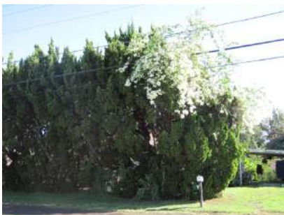
Vegetation overgrowing powerlines is a high hazard
