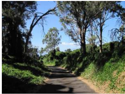
Kealakupu Drive dead tree on roadside and common vines
