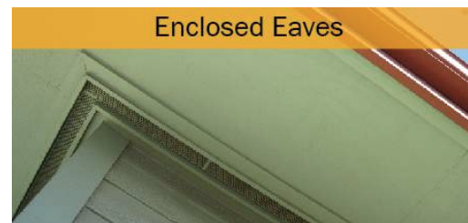
Figure 14. Make sure your eaves are enclosed with non-combustible materials to prevent ember entry.
