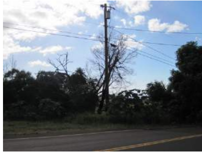
Hwy 37, dead trees near power lines and power poles
