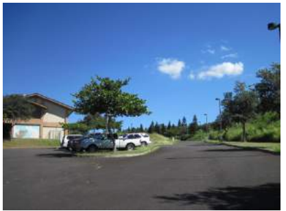
King Kekualike High School adjacent to hazardous tall grassy fuels
