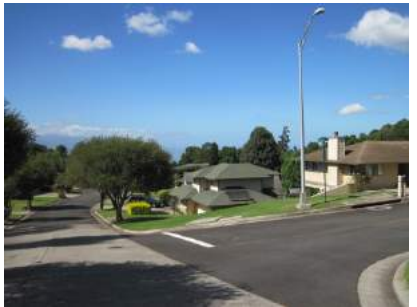
Example of home with low hazard and good access
