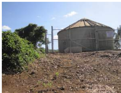
Kealakupu Drive water tank
