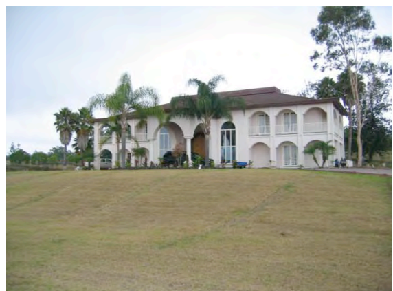
Typical house in Pu'u Lani Ranch Estates. This house has defensible space, although not all homes in the subdivision do.
