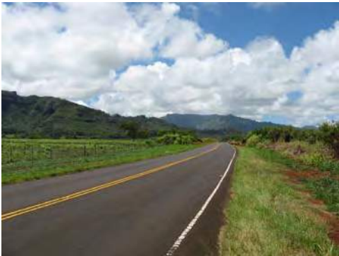
Above: Roadway in Wailua. Collector roads, such as this one, are required to be at least 56 feet wide in accordance with Kauai County Code.
