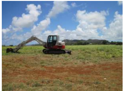
Mechanical treatment to remove fuels along WUI
