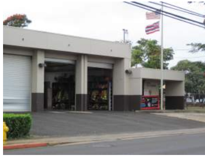
Lihue Fire Station
