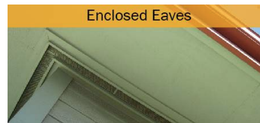
Figure 13. Make sure your eaves are enclosed with non-combustible materials to prevent ember entry.
