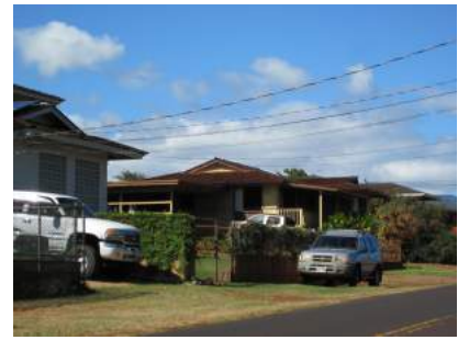
Series of homes with shake roofs
