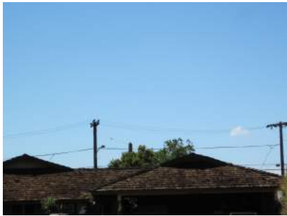
Example of shake roofs
