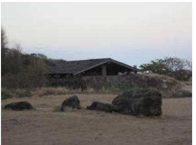
Polihale restroom facilities surrounded by fuels
