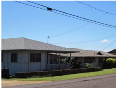
Example of non-combustible roofs
