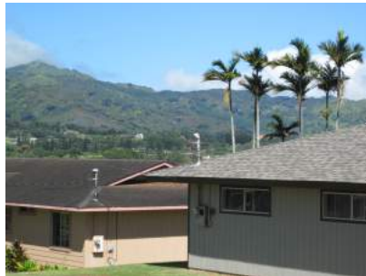
Example of homes with non-combustible roofs and combustible sidings
