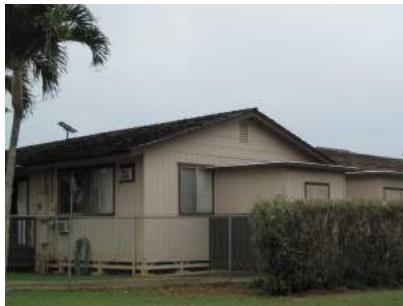
Common shingle roofs and wood sidings in Umi Street neighborhood
