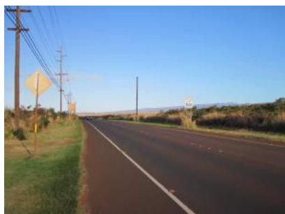
Highway with limited shoulder space
