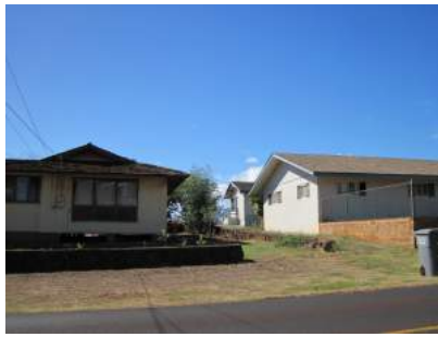
Shake roof home next to hardened home
