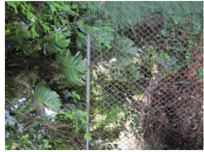
Example of debris piling up along fence line
