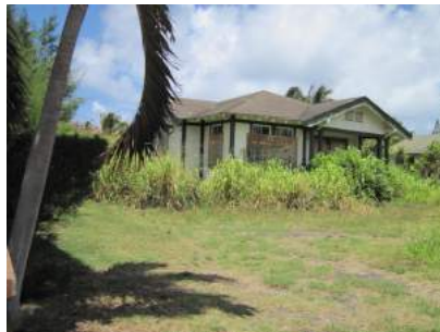
Vacant home with tall grasses surrounding structure
