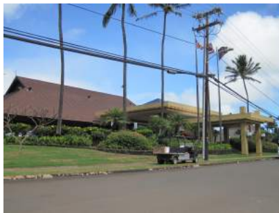
Sheraton Kauai front entrance
