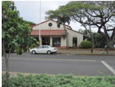
Lihue Post Office with pohinahina in median
