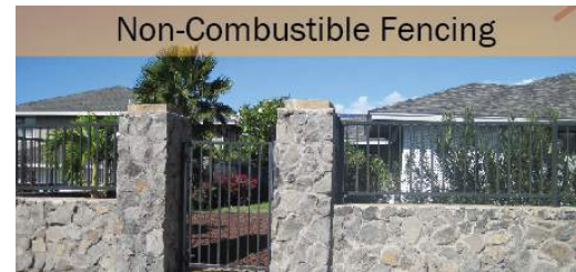
Figure 13. Wood fencing can act like a fire wick straight to a home. Use non-combustible materials for all fencing and yard structures.
