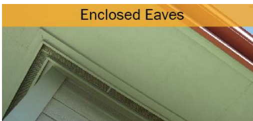
Figure 11. Make sure your eaves are enclosed with non-combustible materials to prevent ember entry.
