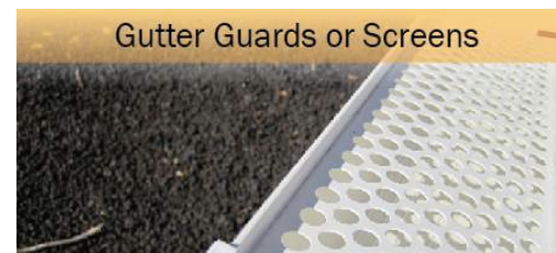
Figure 12. Rain gutters should have screens to keep leaf debris from accumulating. Maintain gutters to keep them clear and clean.
