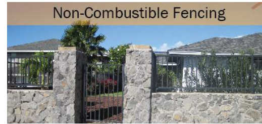
Figure 10. Wood fencing can act like a fire wick straight to a home. Use non-combustible materials for all fencing and yard structures.
