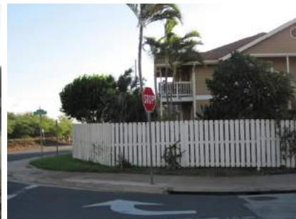
Apartments across from Kenolio fuelbreak area with tall kiawe
