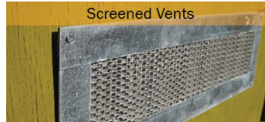
Figure 6. Covering vents with 1/8-inch or smaller metal mesh blocks embers from entering a home or structure.
