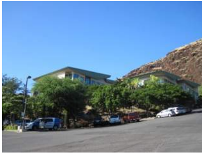
Wai'anae Comprehensive Health Center – entrance to parking lot
