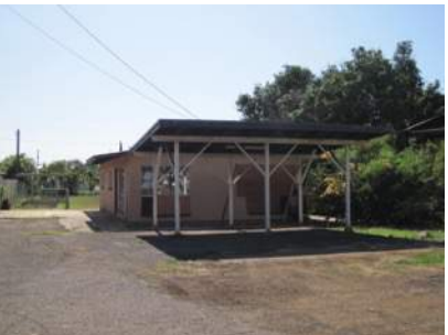
Example of the many vacant homes in the area
