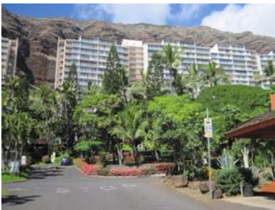
Mākaha Valley Towers
