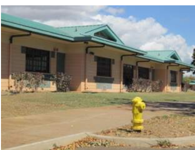
Ho'okele Elementary School with fire hydrant
