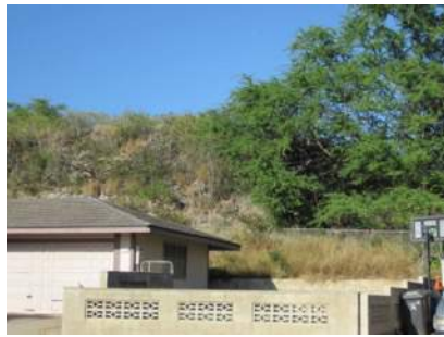
Example of home in Sea Country subdivision with overgrown berm behind structure
