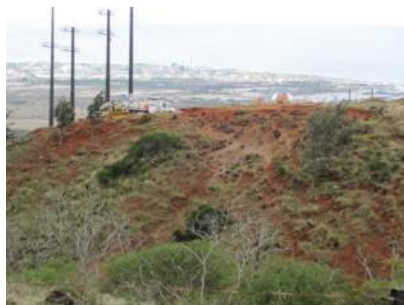
Example of heavy erosion
