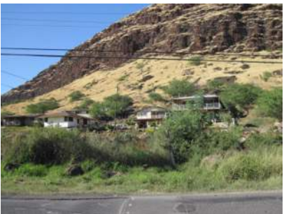
Example of homes surrounded by steep grassy hillside and kiawe
