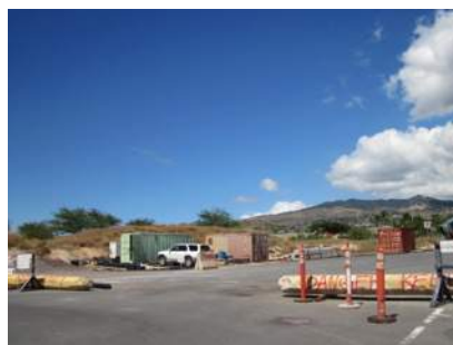
Construction for new Kekala Street development with pockets of unmanaged vegetation
