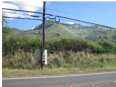
Unmanaged fuels under powerlines along main highway a high ignition risk
