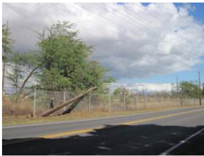
Downed utility pole next to wildland area along FDR Avenue
