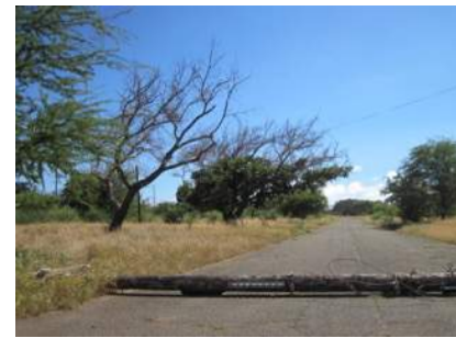
Snags and downed utility pole on decommissioned road off of FDR Avenue
