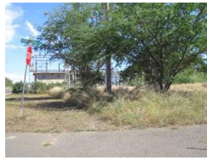
Electric facility surrounded by kiawe and grass along FDR Avenue
