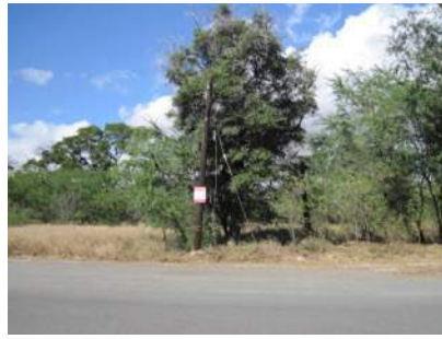
Tall flammable fuels directly adjacent to lamp post on Boxer Road
