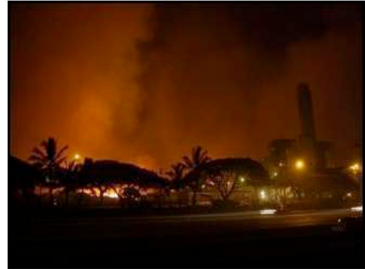
Photo 11. Fire approaches the Hawaiian Electric Co.'s Kahe Point power plant. 3 (Photo credit: Gregory Yamamoto/Honolulu Advertiser).
