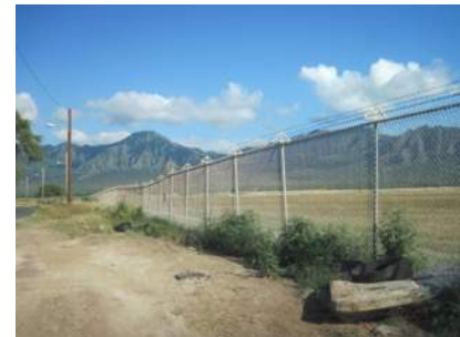
Naval Transmitting Facility along Paakea Road
