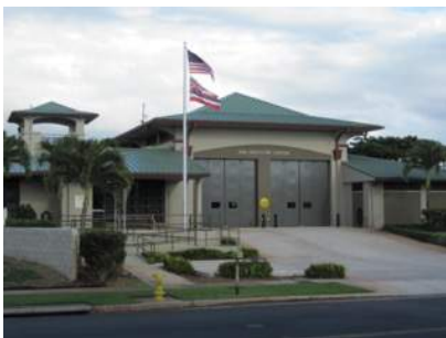
‘Ewa Beach Fire Station
