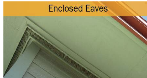
Figure 14. Make sure your eaves are enclosed with non-combustible materials to prevent ember entry.
