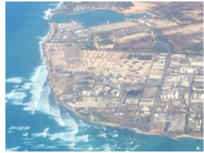
Aerial view of Barber’s Point with large swell
