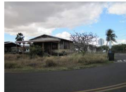
‘Ewa Beach Road – one of a few vacant homes with fuel buildup
