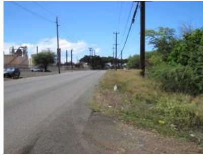
Unmanaged vegetation on road shoulders across from Chevron Refinery
