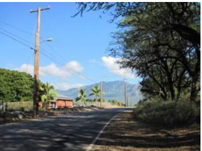
Example of some vegetation management along roadside on Mā'ili'ili Road
