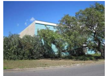
Dense shrubs and trees touching building in Industrial Park
