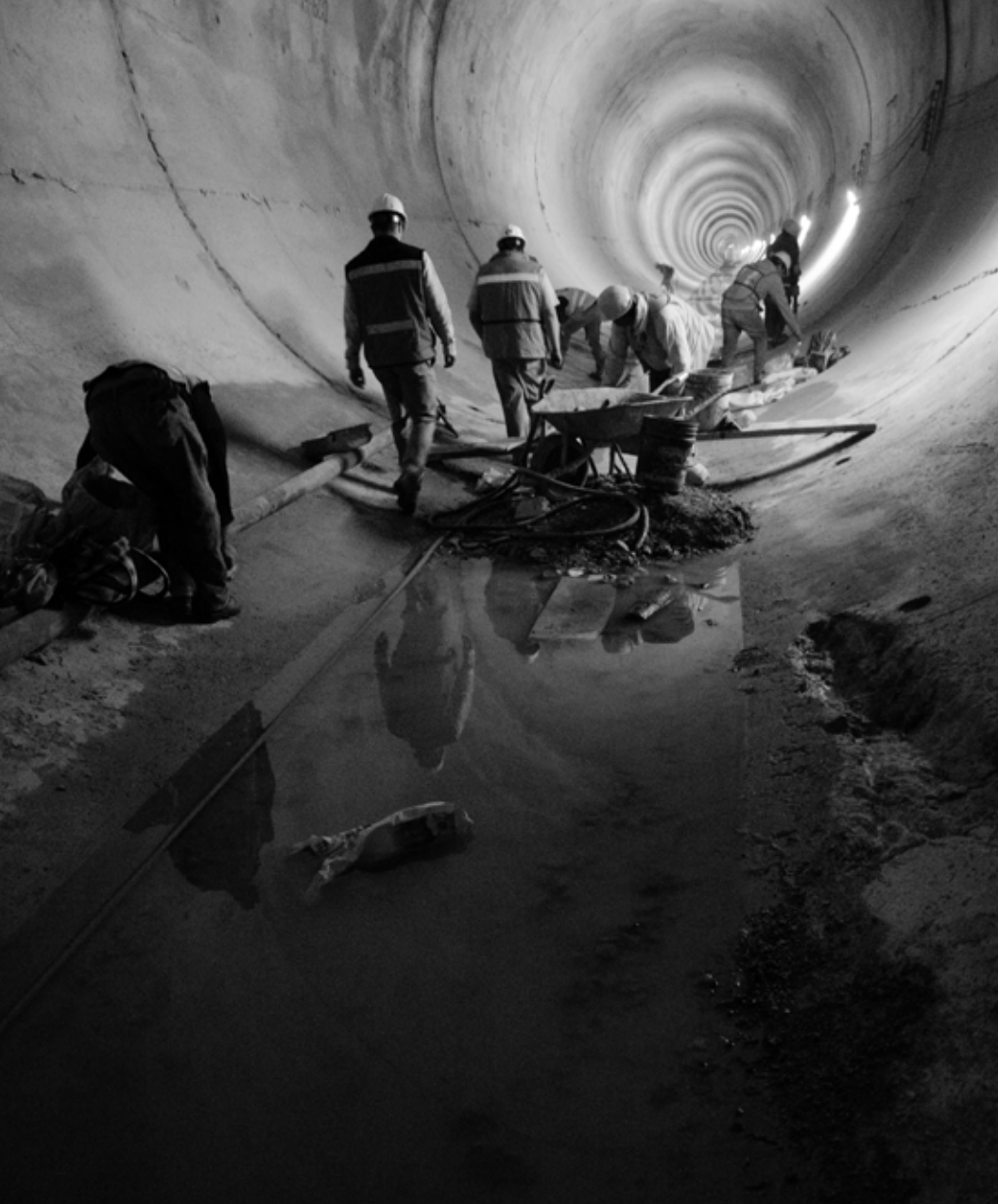
Engineers walking by construction workers in the Eastern Emitter Tunnel.
