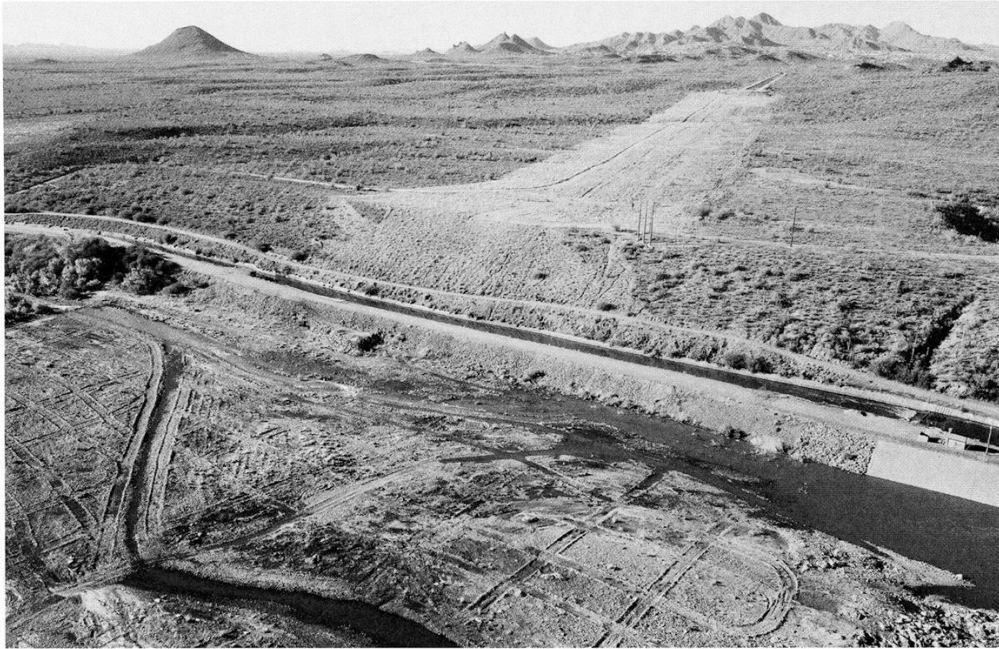
SALT RIVER, GRANITE RIVER DAM AND CENTRAL ARIZONA PROJECT INTERSECTION, MESA, ARIZONA—2007
