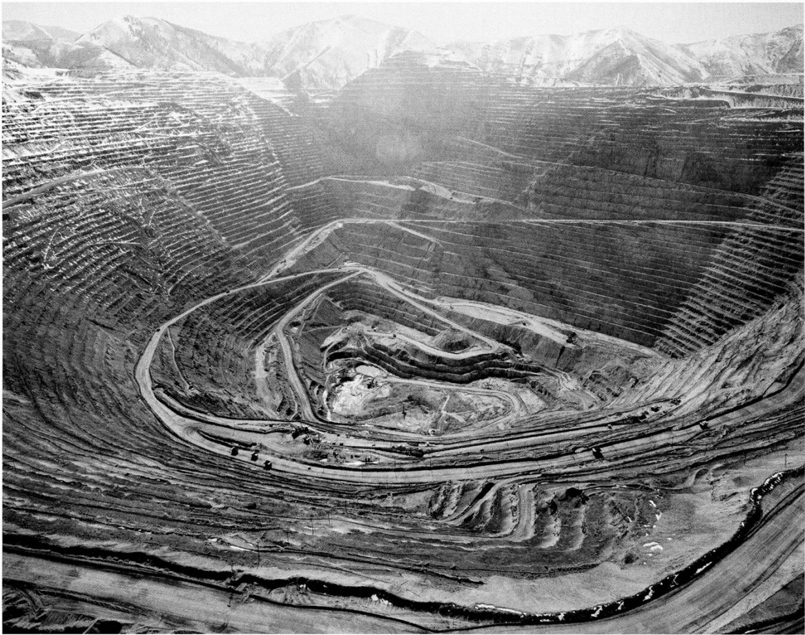
EARTH'S LARGEST EXCAVATION, 2.5 MILES WIDE AND .5 MILES DEEP, LOOKING WEST, BINGHAM CANYON, UTAH—2006
