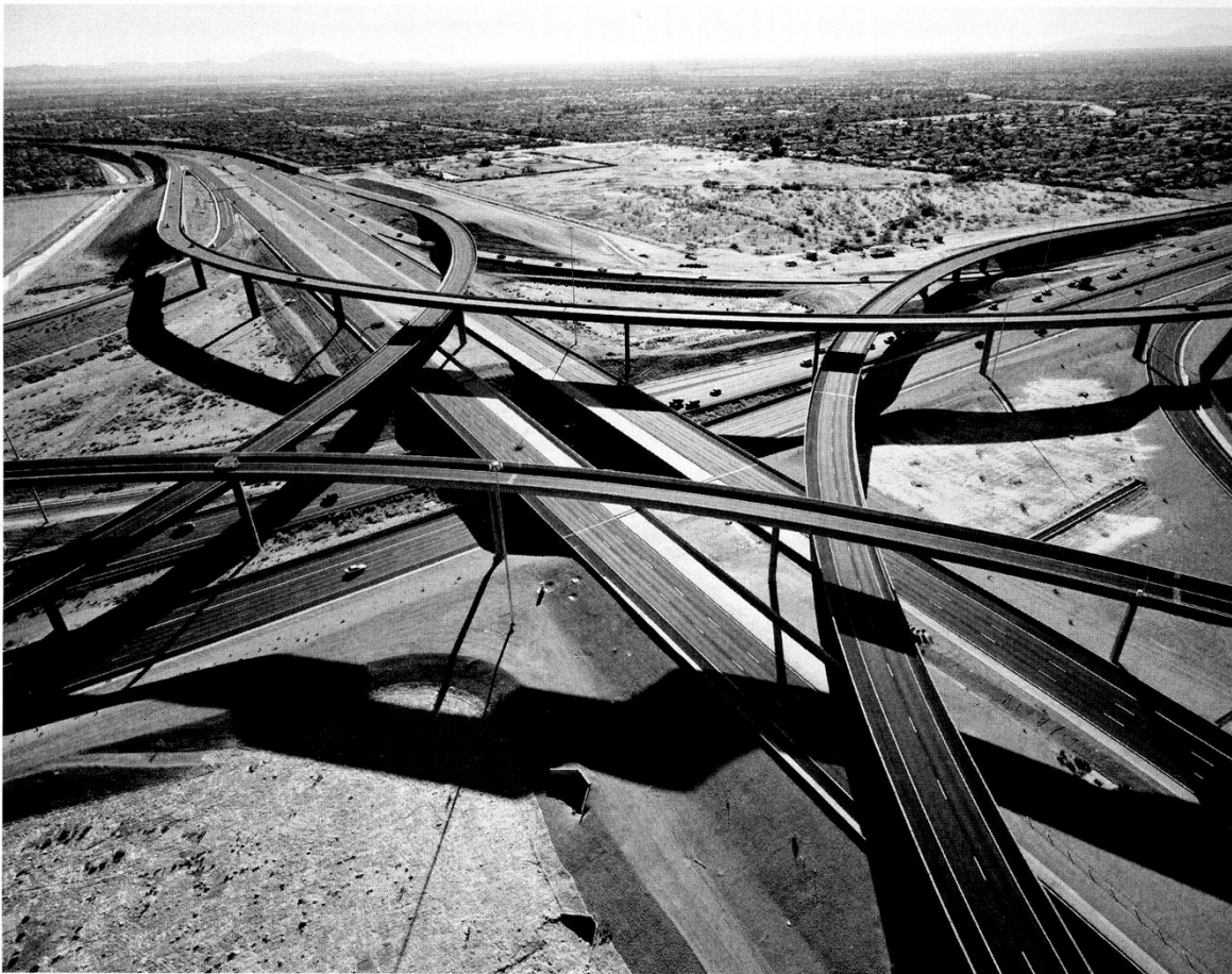
INTERCHANGE OF HIGHWAYS 60 AND 202 LOOKING WEST, MESA, ARIZONA—2007
