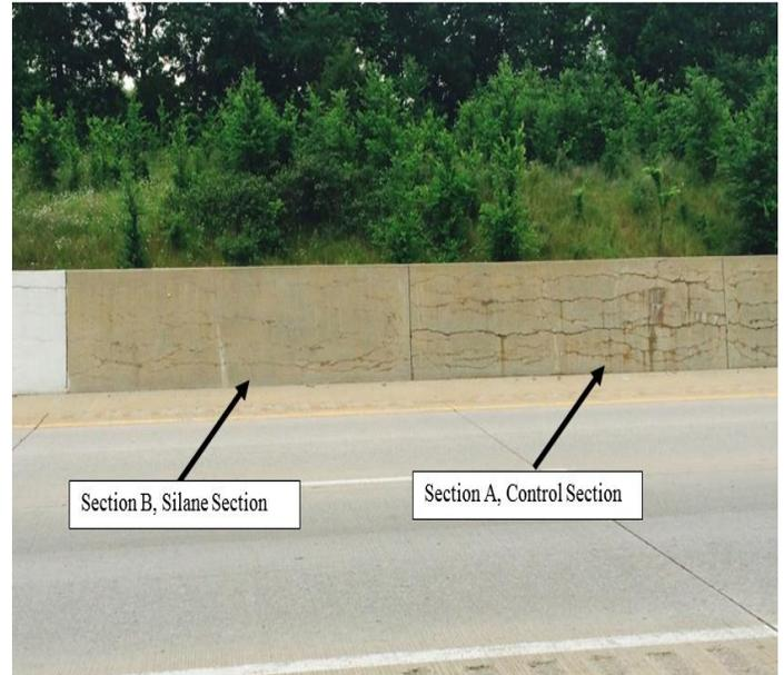
**Figure 4. Barrier Wall Sections**
