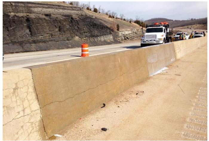
**Figure 1. Moderately Damaged Section of the Barrier Wall Treated with Silane**
