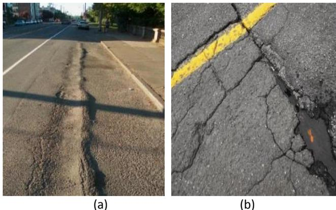
Figure 1: Rutting as a result of Shear Failure and Moisture Damage
