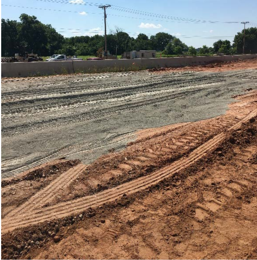
Figure 16. Us-77 Construction Project
