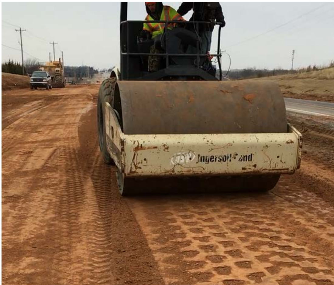
Figure 9. Subgrade compaction on Westbound Hwy-9, Cleveland County, Oklahoma
