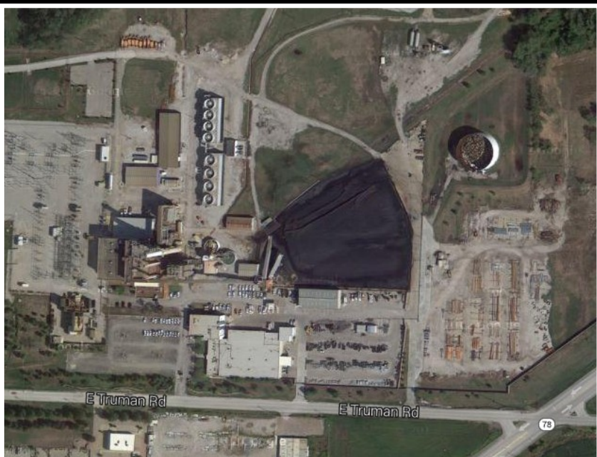
Blue Valley Power Plant
