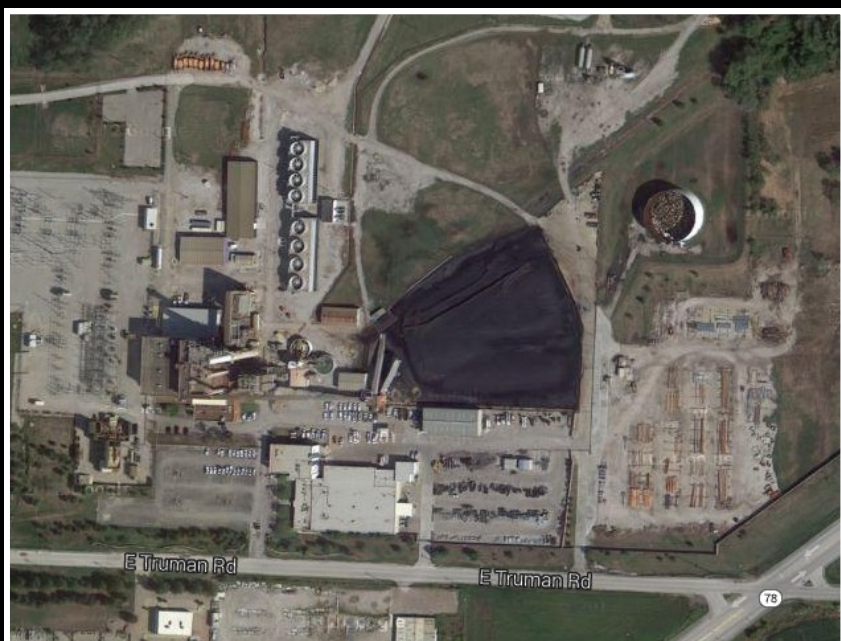
Blue Valley Power Plant
