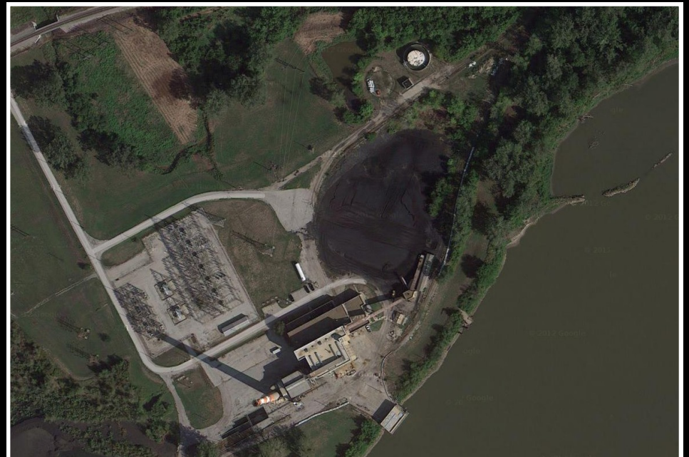
Missouri City Power Plant
