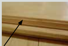
XLplus "nub" provides automatic spacing
