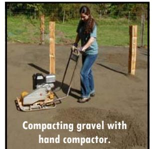
**Compacting gravel with hand compactor.**
