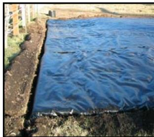
**Geotextile fabric installed on bare ground and tucked into trench.**
