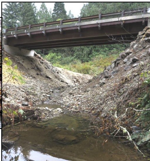
After: 50 foot span bridge to allow proper fish passage.
