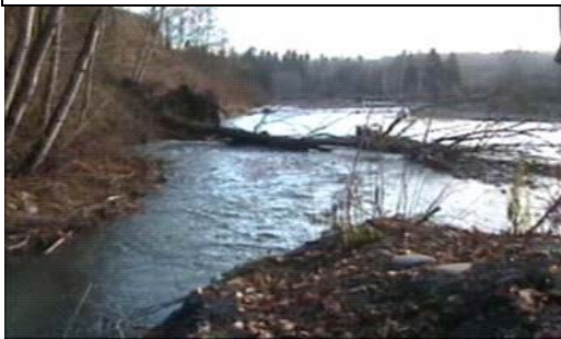
Exhibit 2-33 Independent Canal Intake Channel at Dungeness River
