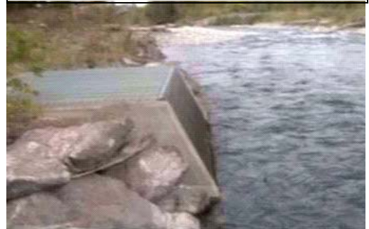
Exhibit 2-23 CCD Intake Structure
