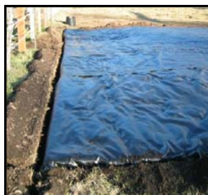
Geotextile fabric installed on bare ground and tucked into trench.
