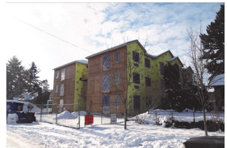
Under Construction 18 Unit N Minnesota Apartments 6195 N Minnesota Ave, Portland
