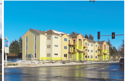
Under Construction 24 Unit Sierra Point Apartments 3359 SE Powell Valley Road, Gresham
