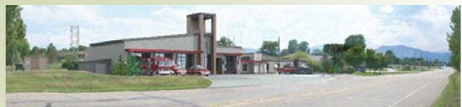
Rocky Mountain Fire Station #1, Boulder OZ Architecture Anticipated completion: September 2012
